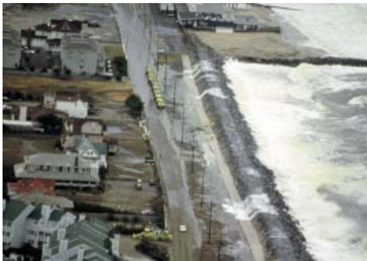
View of Sea Bright, New Jersey, coastline as a storm attacks the seawall.
