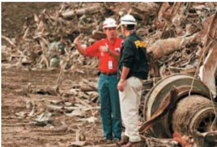
Staten Island, New York, October 16, 2001. David Leach of the Army Corps of Engineers explains to Ted Monette, FEMA federal coordinating officer, the process for handling debris being removed from Ground Zero to the landfill. By mid-October 2001, approximately 10 ton of debris were being processed daily for evidence related to the attack. (Photo by Andrea Booher/FEMA News photo)
