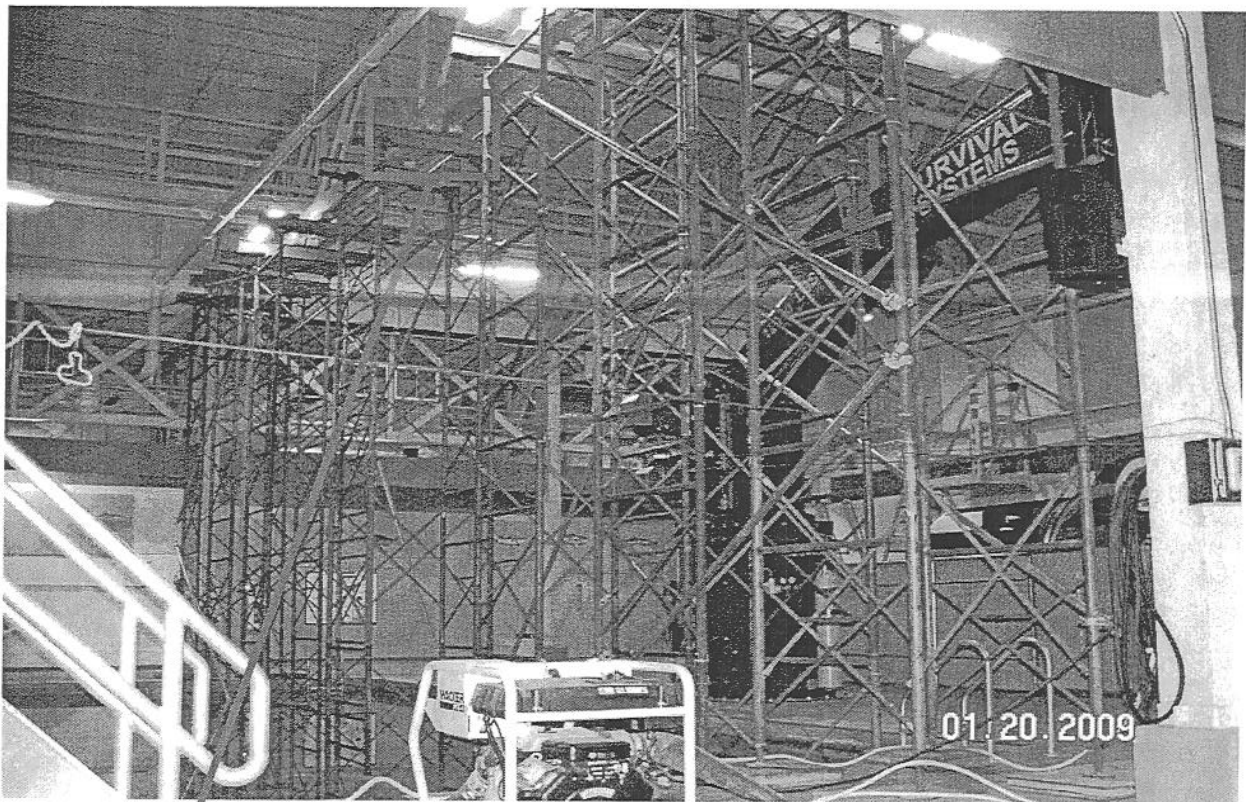
Picture 2: Bracing used to stabilize SERE pool roof during snow loading
