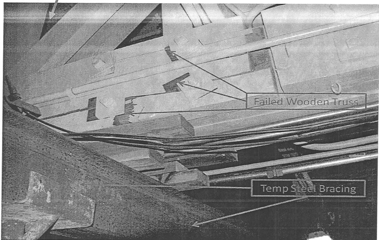
Picture 3: Example of a failing wooden truss, being supported by temp steel bracing
