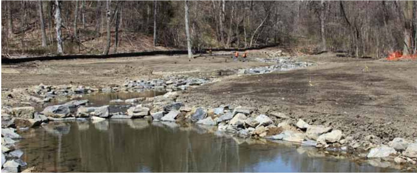
Touring the project site at Indian Creek, a tributary of the Cobbs Creek watershed. The project is designed to reduce combined sewage overflow and improve habitat. (Photo by USACE Philadelphia District & Marine Design Center)
