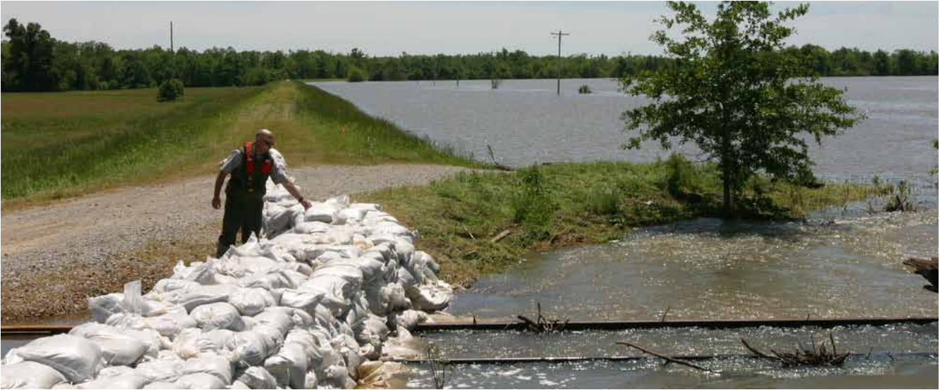
An Army Corps of Engineers Natural Resource Specialist inspects levees between Jacksonport and Newport, AR. (Photo by Laurie Driver)
