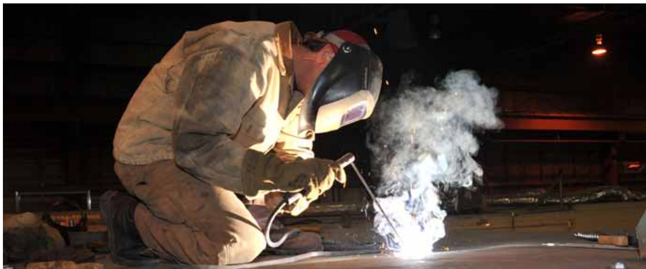
A welder working at Ensley Engineer Yard. (Photo by Stacy Ouellette)
