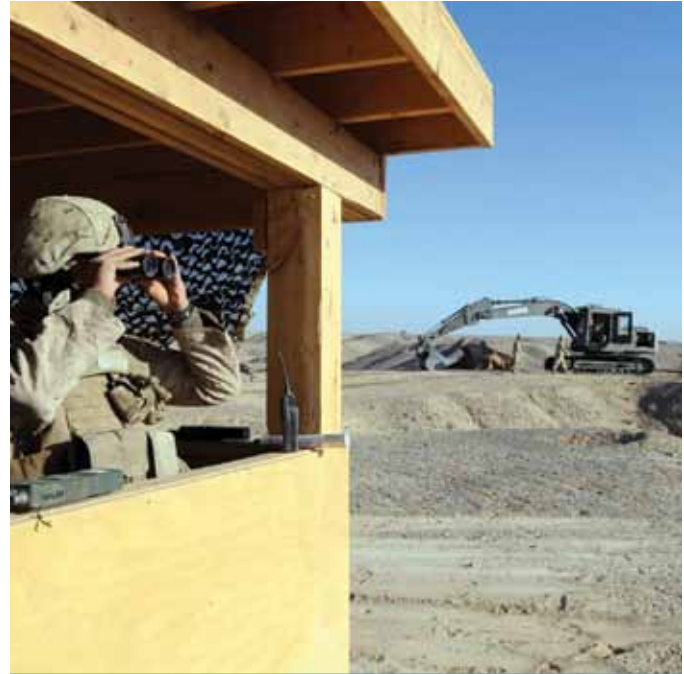
A Lance Corporal assigned to Marine Corps 3rd Light Armored Reconnaissance Battalion (3rd LAR) stands watch as Seabees assigned to Naval Mobile Construction Battalion (NMCB) 3 prepare a look-out post at Forward Operating Base Payne, Helmand Province, Afghanistan.
