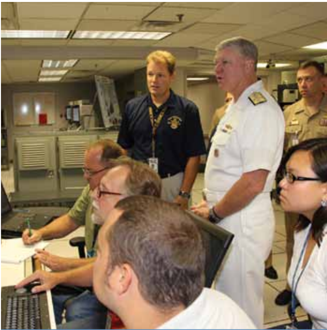
Chief of Naval Operations, Admiral Gary Roughead, views components of the DDG 1000 Integrated Power System land-based test site on board Naval Surface Warfare Center Carderock Division, Ship Systems Engineering Station, Philadelphia.
