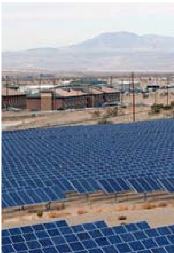
Solar panels supply energy to Marine Corps Air Ground Combat Center. Twentynine Palms, California – February 2009
