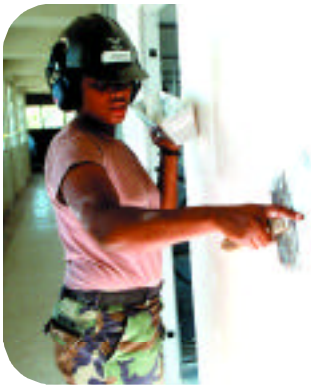
A builder 3rd Class plasters a wall inside the Bundy Barracks at NAS Roosevelt Roads, Puerto Rico.
