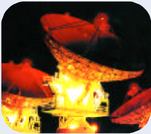
A view of the satellite dish arrays at the Naval Computer and Telecommunications Area Master Station in Honolulu, HI.
